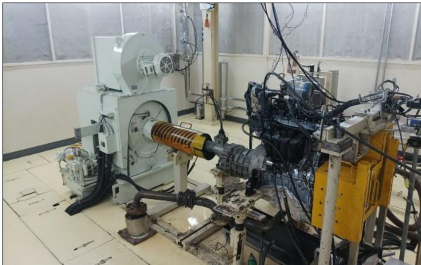
Figure 2. Engine Dynamometer Installation
